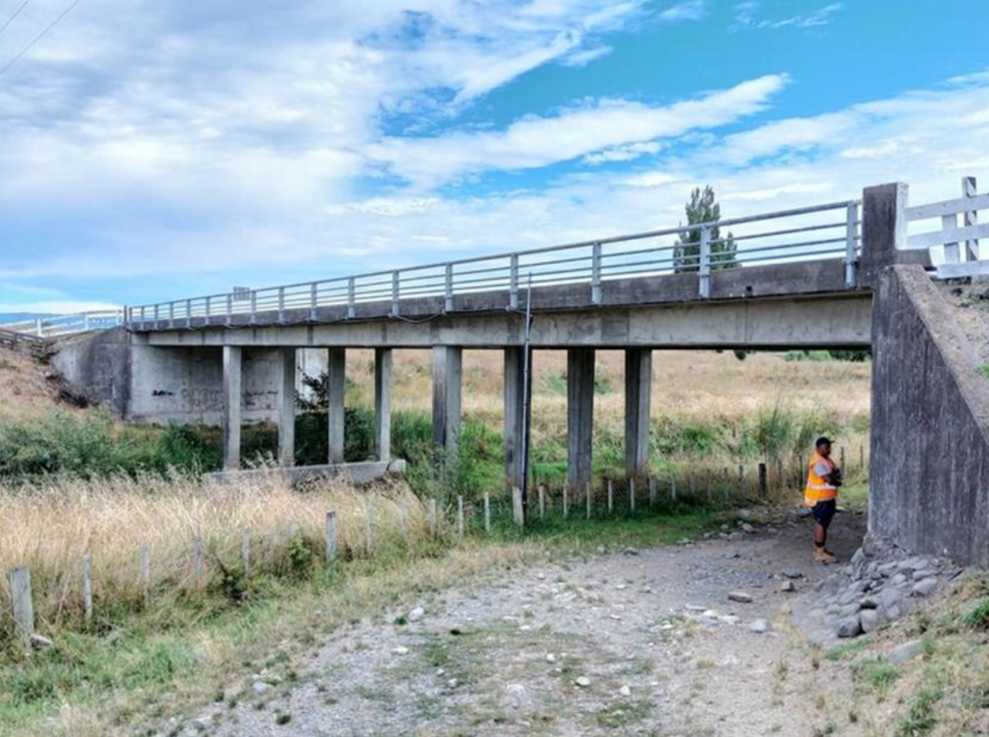
Photo: 37.2m Concrete bridge built in 1955.
