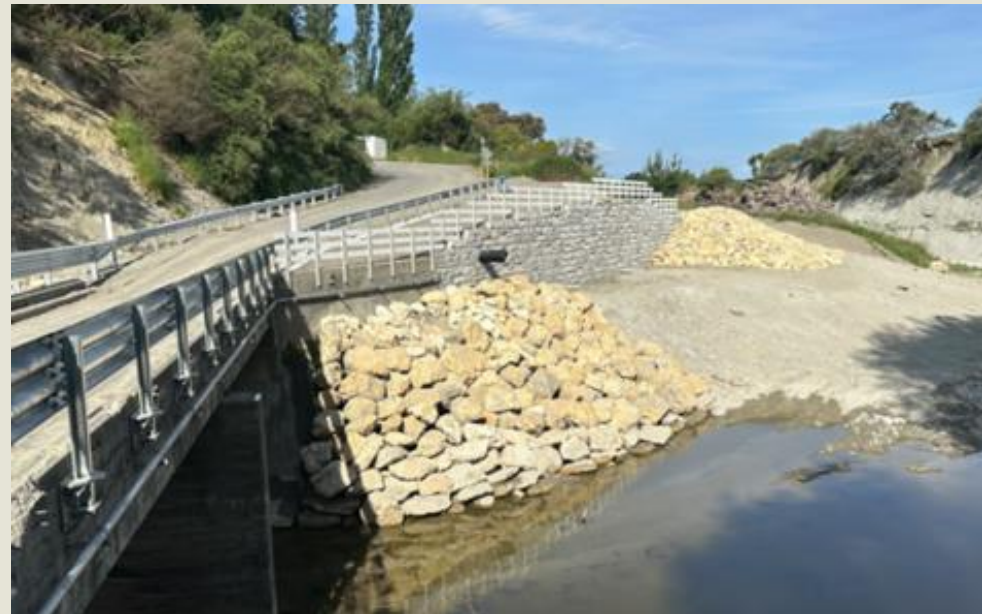
Crownthorpe Bridge, before and after repairs.
