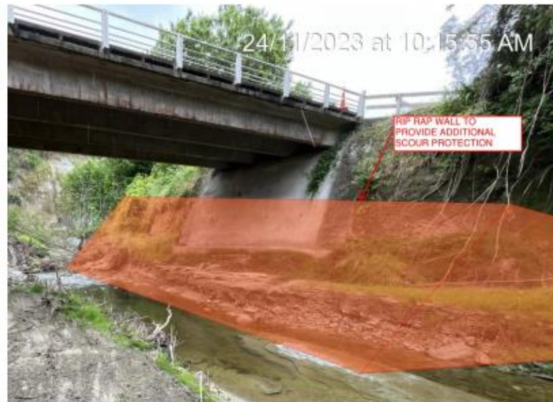
Figure 6-1: Indicative sketch showing rip rap wall at the eastern bridge abutment for additional scour protection.
